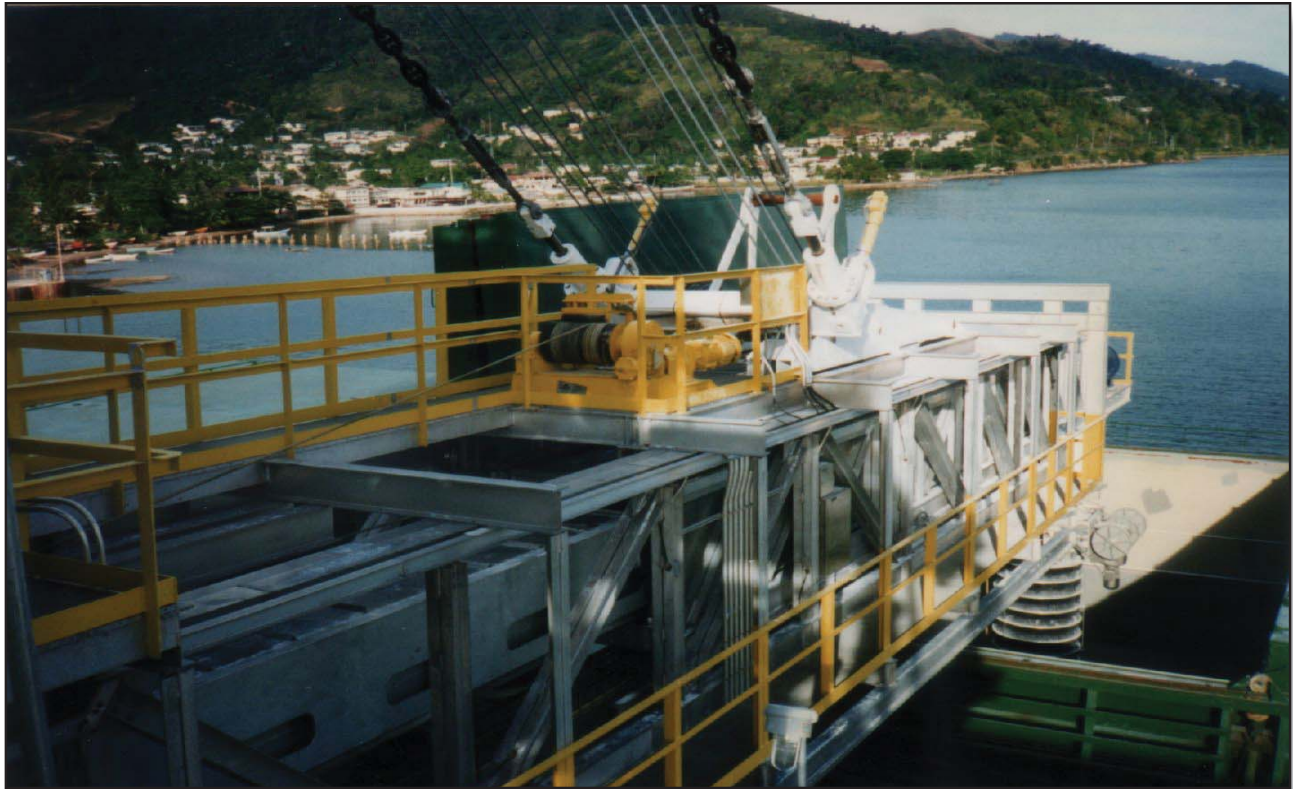
Example of shiploading with new equipment
