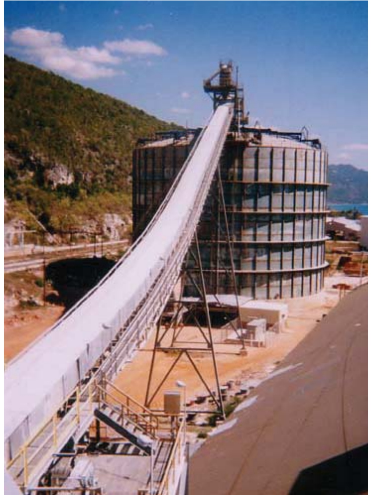
Silo & Feed Conveyor
